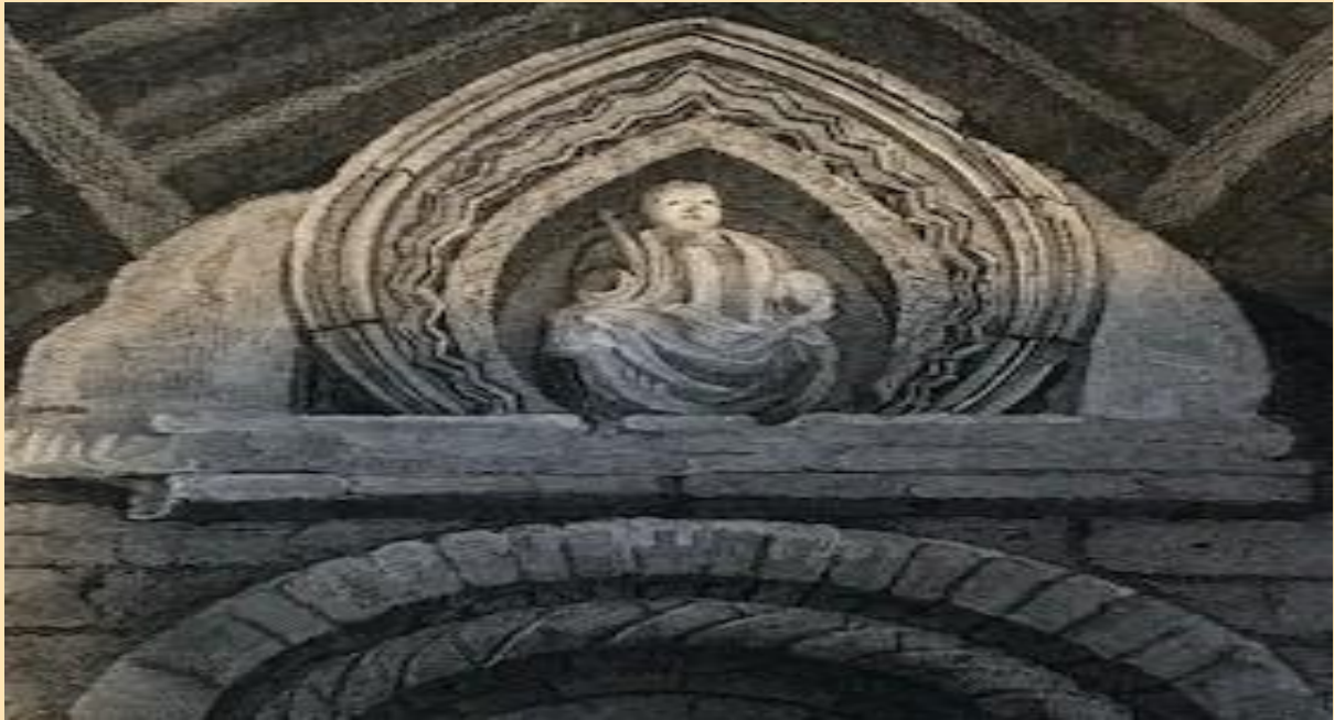
Above – The 1815 Engraving of St. Nicholas? Note- The Vesica at that time was surrounded by a wooden canopy.
