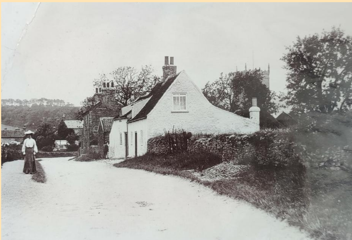
Two cottages (now demolished) on land now occupied by No. 11 South Newbald Road
